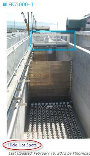
Figure 2.27 Hot Spots Visible
