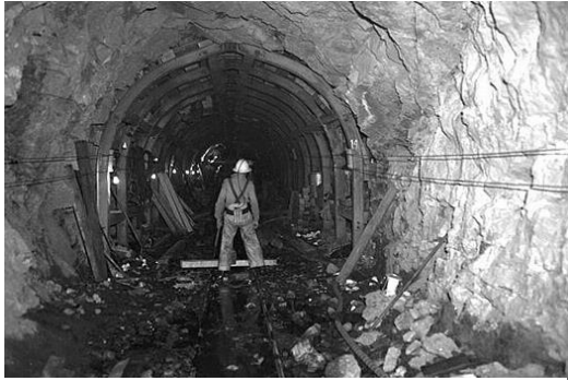
Roberts Tunnel construction
