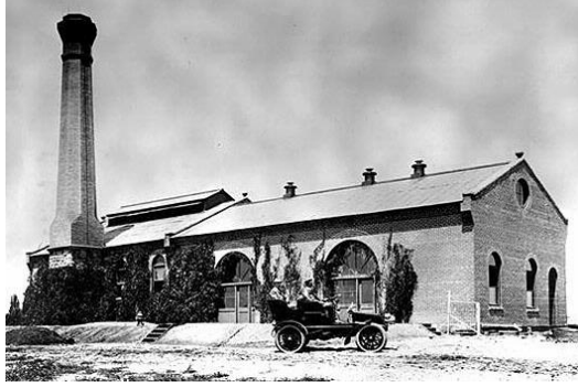
Capitol Hill Pump Station 1905
