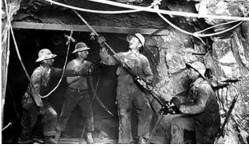
Crews working on Moffat Tunnel October, 1932
