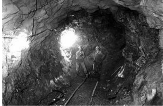
Gross Reservoir construction, Aug. 30, 1951
