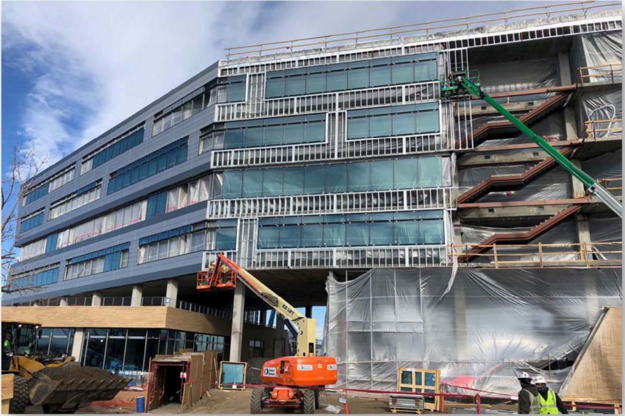
Administration Building irresistible stair and exterior enclosure along south elevation
