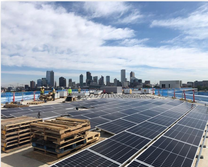
Solar Panel installation Administration Building
